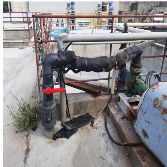
污水接管截止阀
