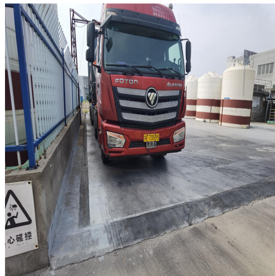
废酸装卸区围堰
